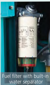
Pre-fuel filter with built-in water separator
